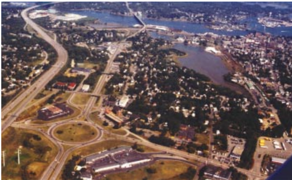
Figure 6 Aerial view showing the flow of Hodgson Brook to the North Mill Pond and the Piscataqua River.
