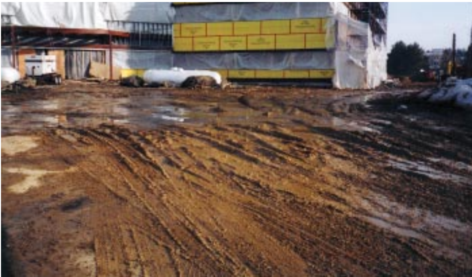
Figure 10 Construction projects as a source of sediment runoff.
