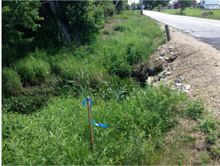
Site 3: On Dudley Brook upstream of North Road culvert just east of the Rockingham County Complex; access from North Road.
