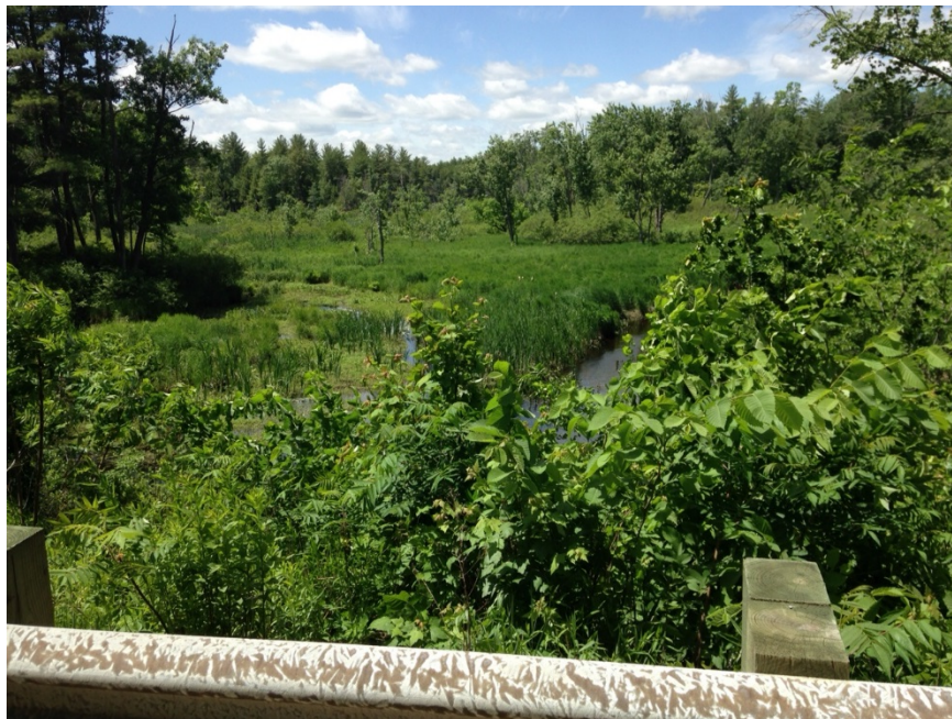
Site 4: On Dudley Brook on the upstream side of the Pickpocket Road culvert; sample taken from directly upstream of culvert; access from Pickpocket Rd.
