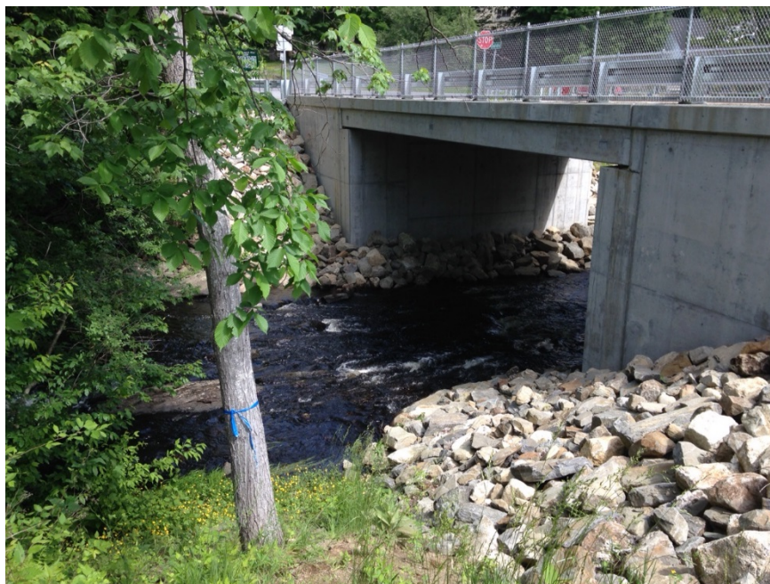
Site 8: On Exeter River between Route 125 Bridge and Crawley Falls Rd. Bridge (shown here); access from Crawley Falls Rd.
