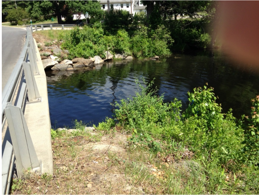
Site 7: On Exeter River on downstream side Route 107 Bridge (shown here); access from Route 107.
