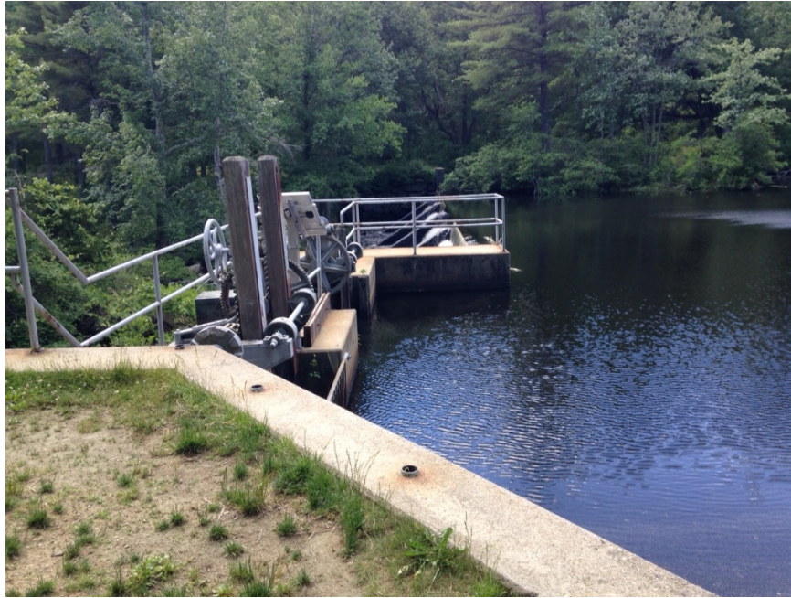
Site 14-EXT: On Exeter River just above the first Pickpocket Dam; sample was taken from cement structure closest to the dam flow; access from Cross Rd.
