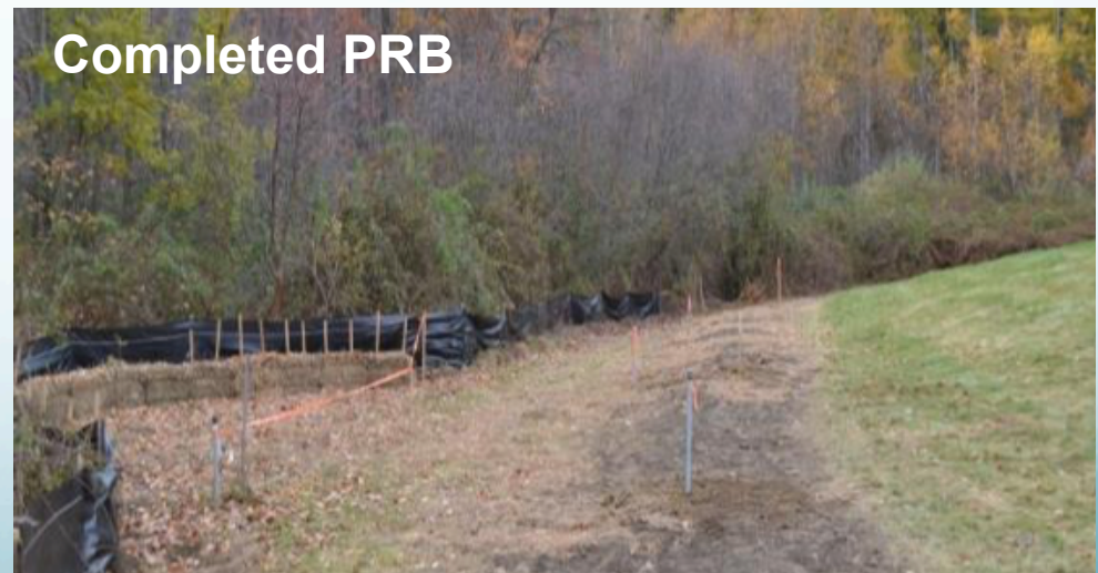
Geotextile cover at surface of trench
