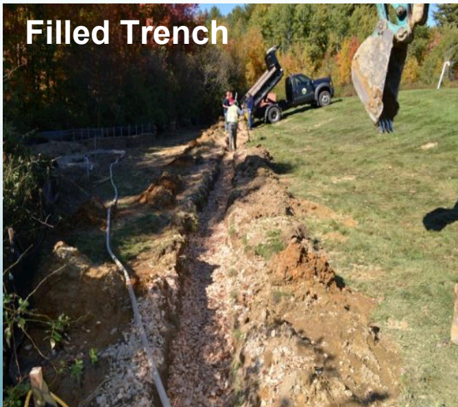
Filling trench with chips as trench is excavated
